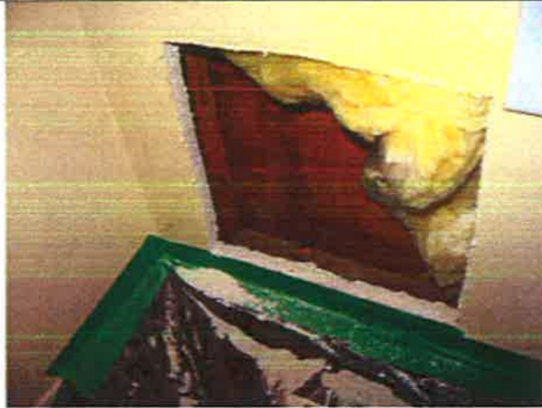
Photo 7: Unit 108 – Interior exploratory opening
