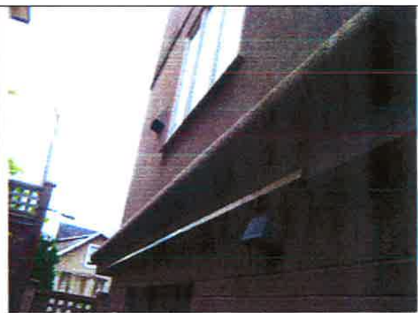
Photo 2: Unit 206 – Localized rehabilitation of the EIFS band
