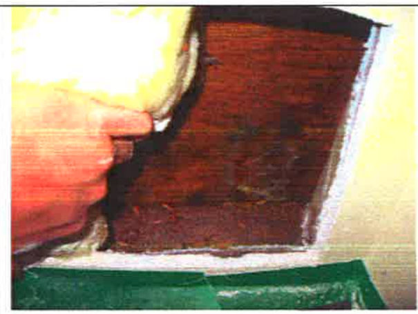
Photo 4: Unit 103 – Interior exploratory opening
